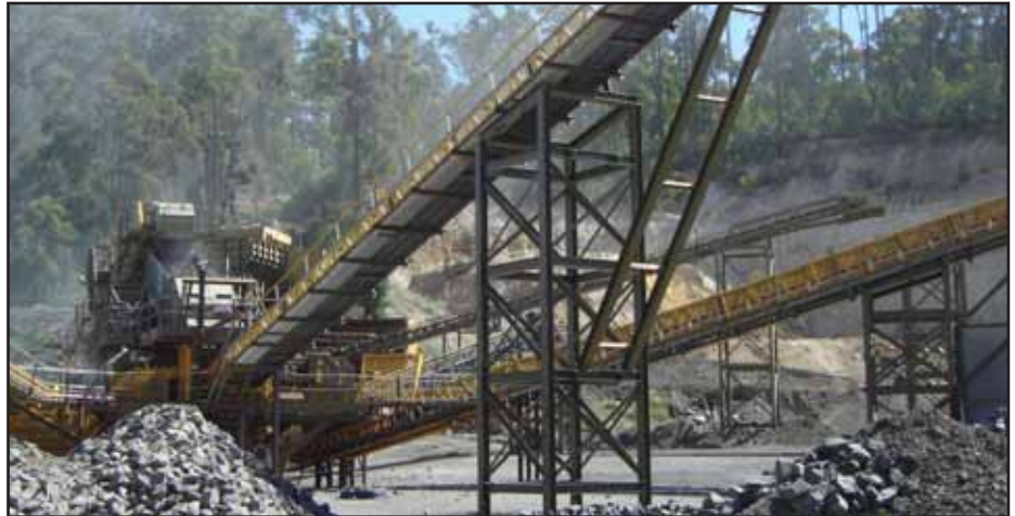
Site Photo – K & RJ Matthews Quarries
