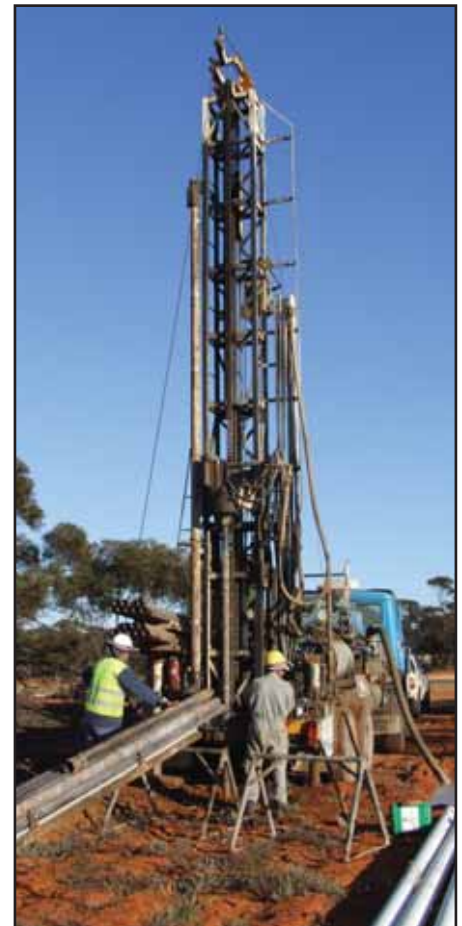
Drilling for groundwater
