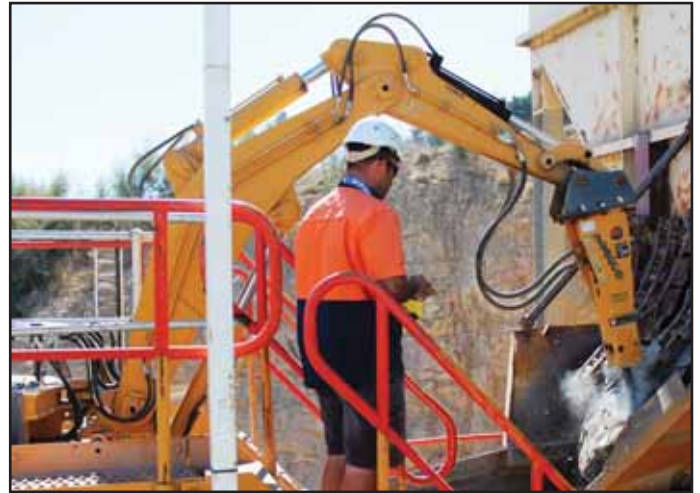
The Indeco HP 200 makes light work of a large obstruction
