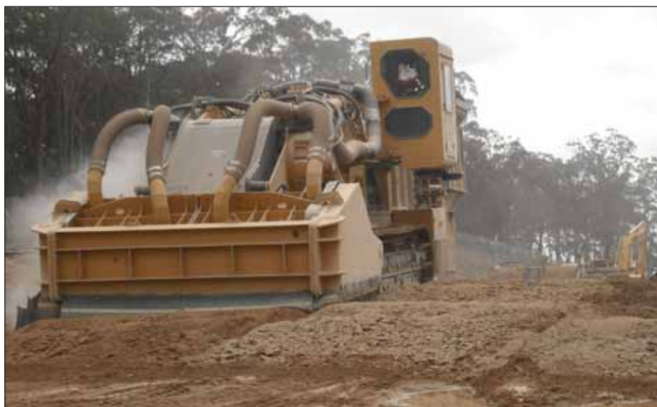
Vermeer T1255 Terrain Leveller working on the Eastern Section
