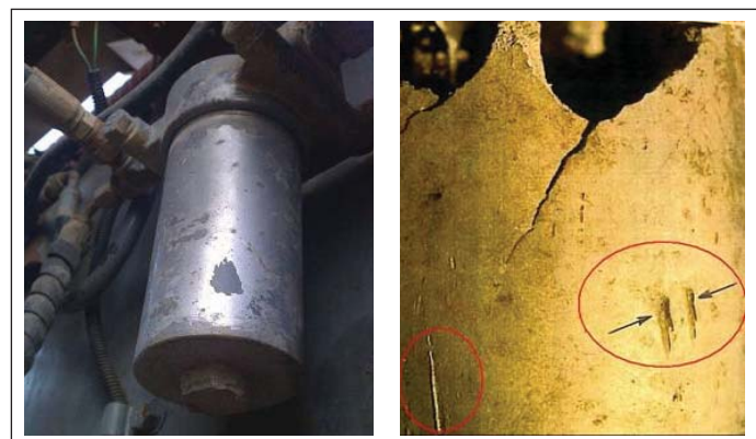
Photo 3 – Stilson marks and cracks on filter housing
