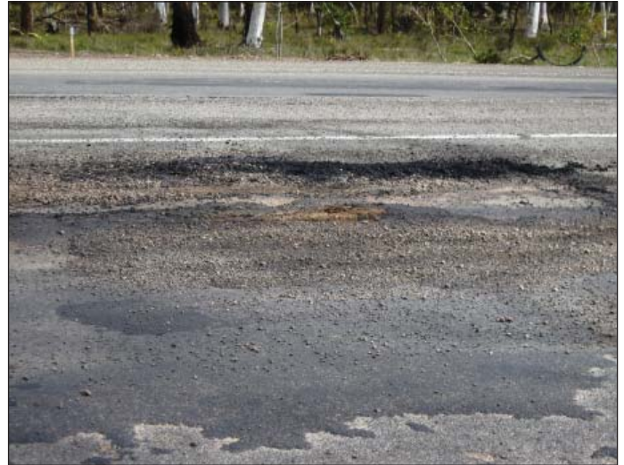
Major pavement failure of recently constructed works on a major state highway in Victoria
