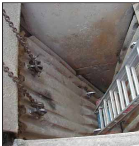
Jaw liner in place
