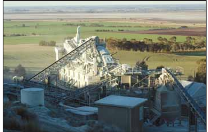
Site Photo – E B Mawsons & Sons Pty Ltd's site Lake Cooper
