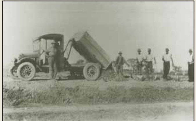
Mawson's road building team, Murray Valley Highway 1930
