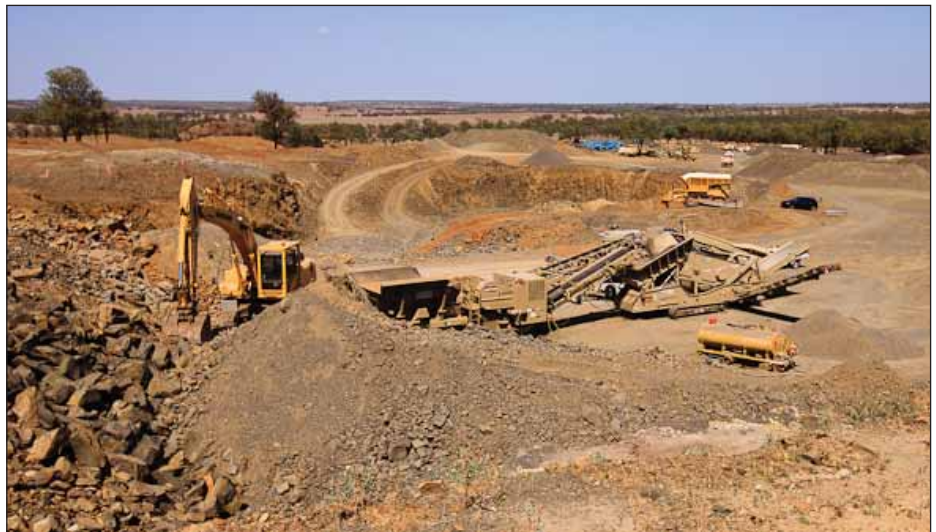
Site Photo – Roma Quarry
