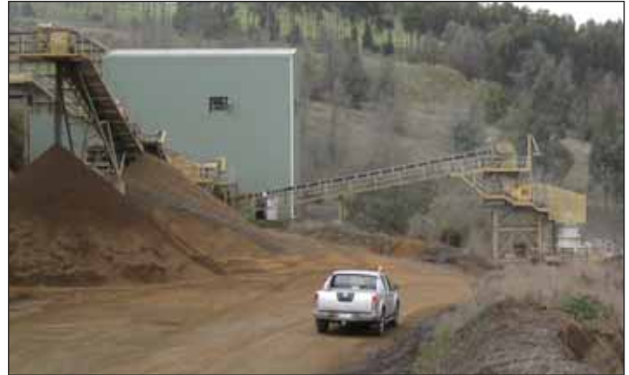
Site Photo – Galli Quarries
