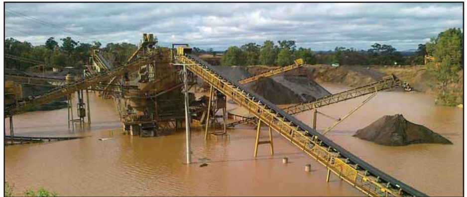
Site photo demonstrating the effects of heavy rain
