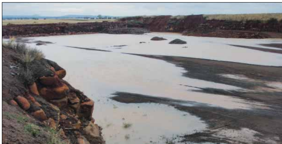
Flood water in a quarry. May not always be a problem if it supplements a quarry's water supply and the water can be saved to an appropriate storage
