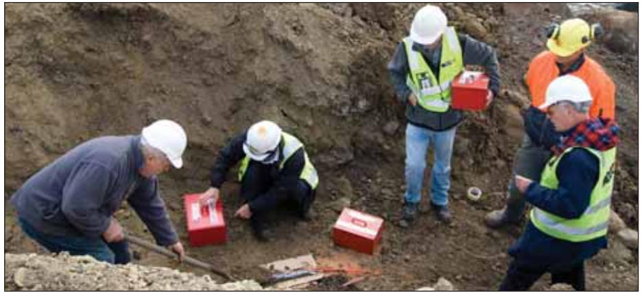
Preparation for shot firing
