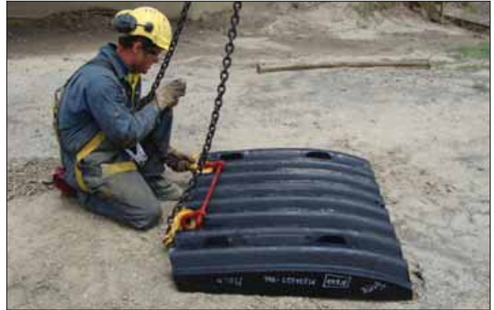
Installation of Mangasafe to jaw liners
