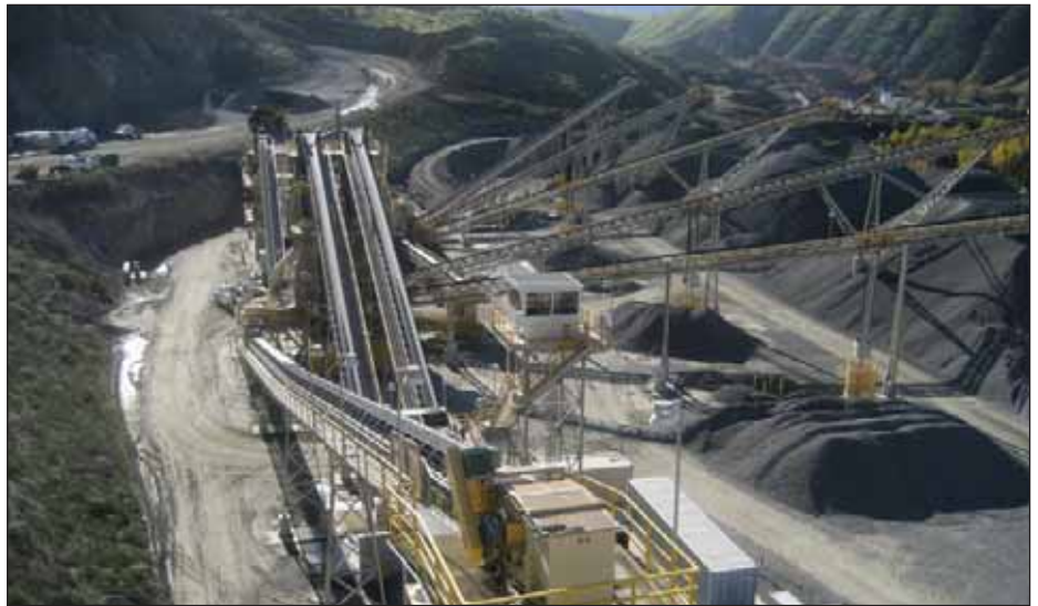
Conveying downhill to reduce electricity costs
