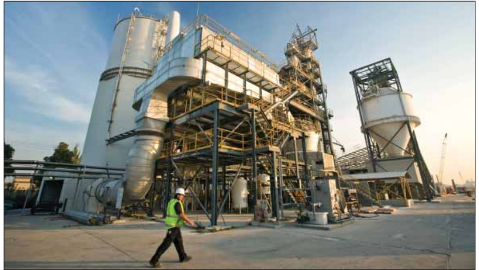
Site Photo – Steel Cement grinding mill
