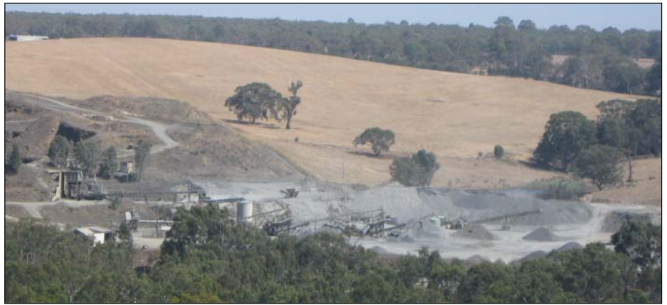
Site photo – Moree Quarries
