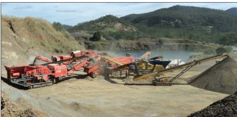
Site Photo – Finlay Screening & Crushing Systems at Gladstone, QLD
