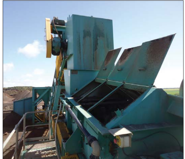
Open Pugmill ready for inspection
